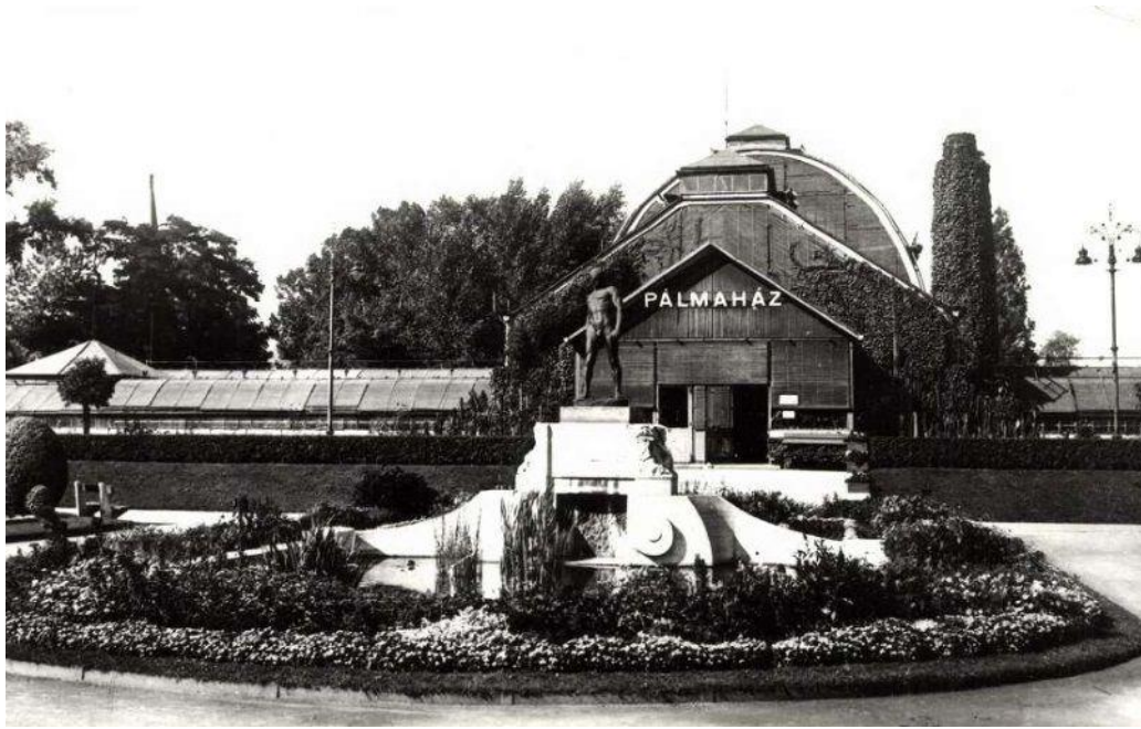
Figure 38. Budapest palm house with geothermal heating [17]
