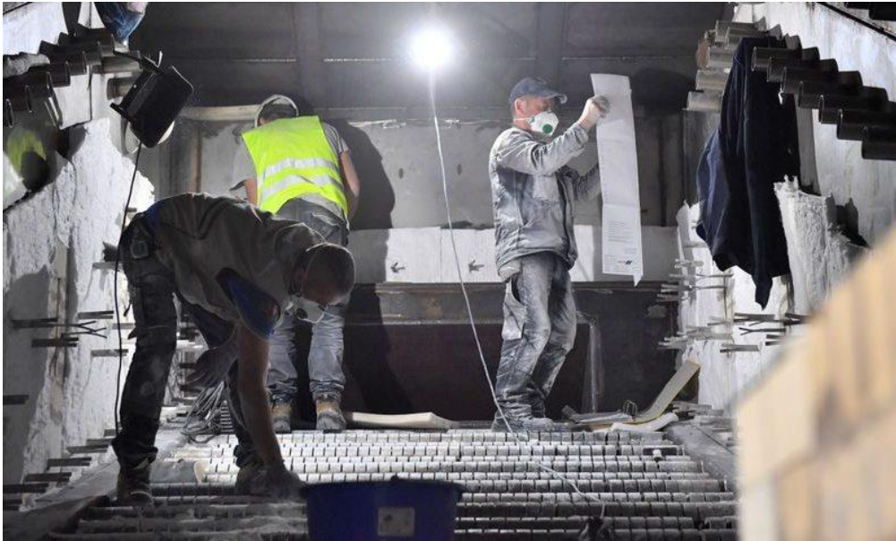
Figure 9. Step grate boiler (7.5 MW) under construction [9]
