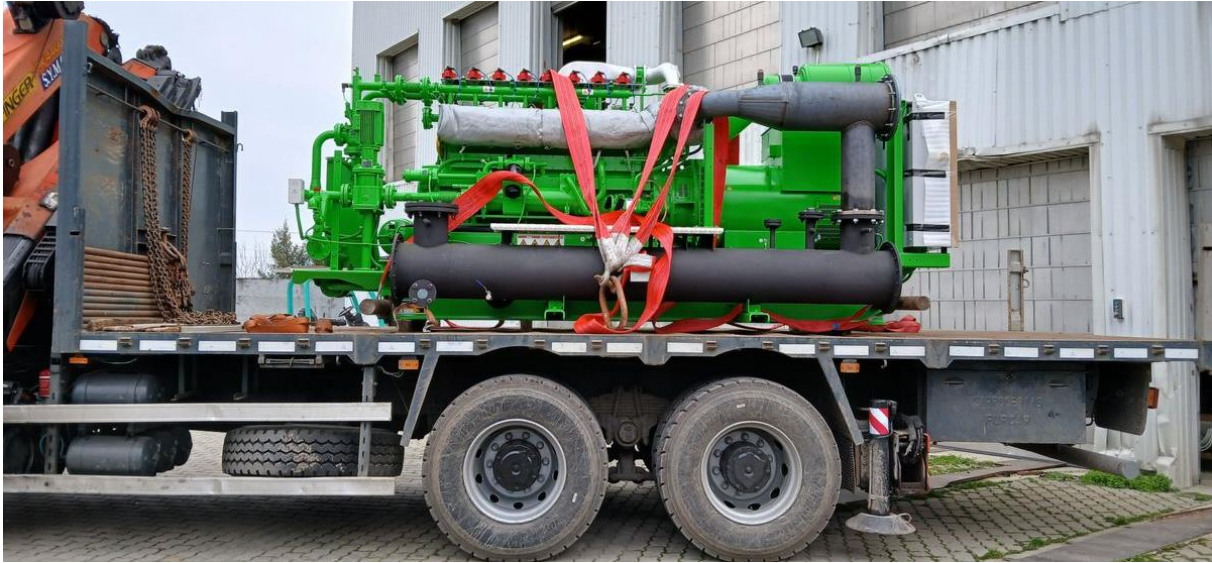
Figure 17. Biogas engine installation [14]
