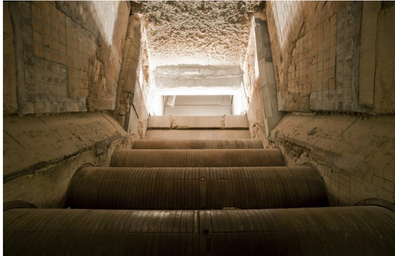
Figure 11. Rotating grate (40 MW) under maintenance [10]
