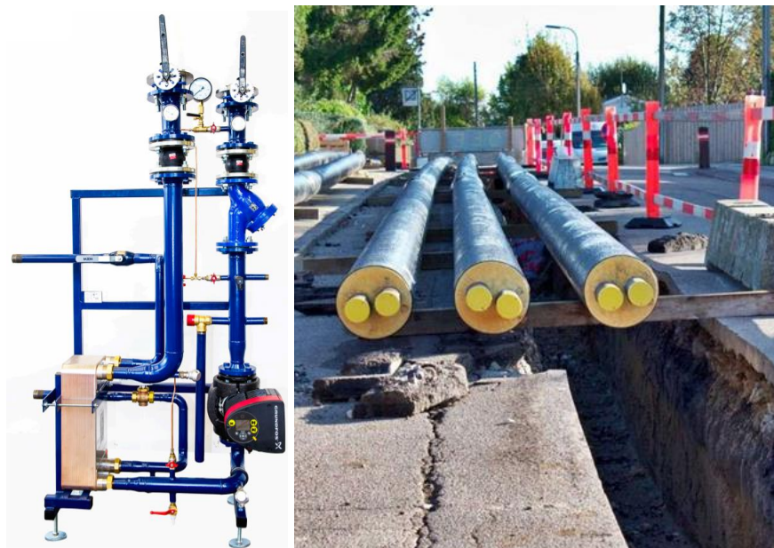
Figure 8. Prefabricated modular DH substation (left) (fotavhu), pre-insulated piping (right) (magyarepitok)
