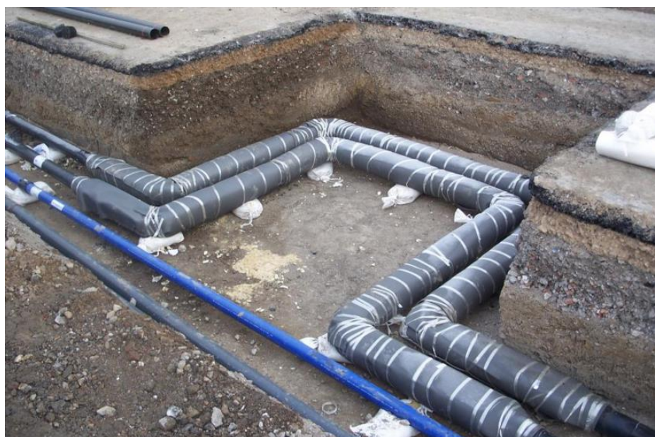
Figure 7. Underground DH pipelines with U-bends compensate thermal expansion [15]
