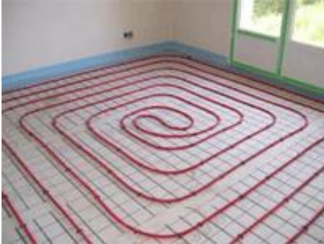
Figure 34 Example of a heating floor
